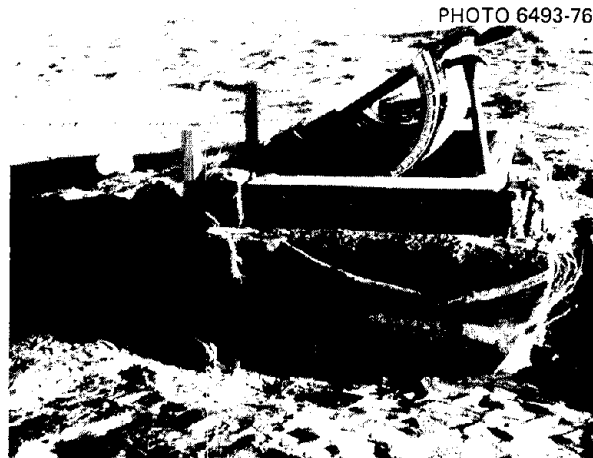
Fig. 7.1. Semiexpedient blast door made of a 30-gal steel drum, badly damaged at 31 psi but still blast-tight. Blast-wind scouring had removed up to 17 in. of the dry earth mounded around this entrance and blown away its single blast-protector log.
